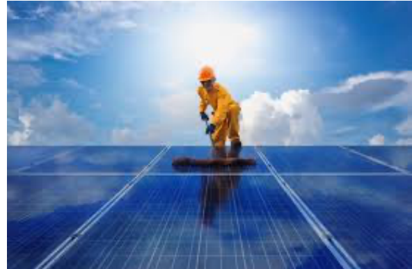
Figure 6: Cleaning solar panels
